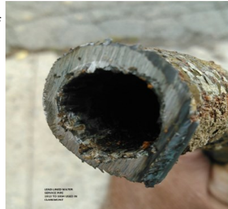
Lead-lined Service Pipe Claremont, NH 1912-1934
