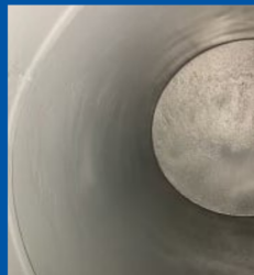
AFTER (with liner)
