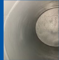
AFTER (with liner)
